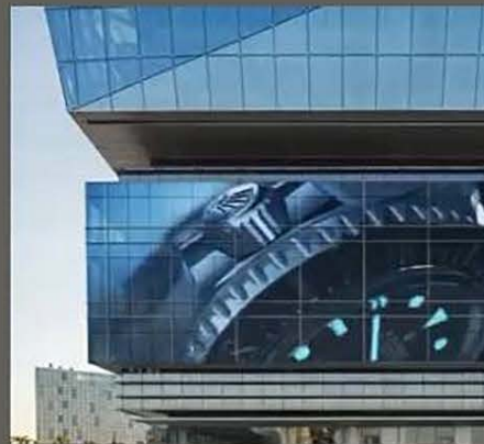
Glass Curtain Wall
